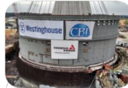
Construction and module assembly
